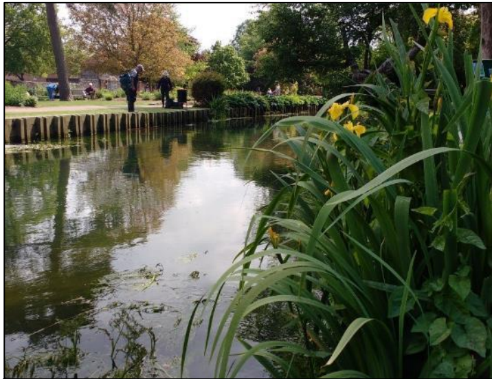
Planting pockets along the edge of a river revetment , Westgate Gardens Canterbury, Kentish Stour Countryside Project
